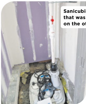
The second Sanicubic 2VX was installed for two side-by-side restrooms, also receiving wastewater from the first Sanicubic 2VX. All the wastewater within this second unit discharges into the conventional plumbing system of the pre-existing restrooms.
