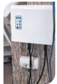
The control panel has a visual and audible alarm system (including a 15' wire).
